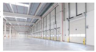
The building has a BACACIER metal roof with a TPO waterproofing membrane and facades made of sandwich panels with a U-value of 0.30 W/m2K and prefabricated thermal break panels with a U-value of 0.34 W/m2K. The complex also includes two battery charging rooms and a guard room.
